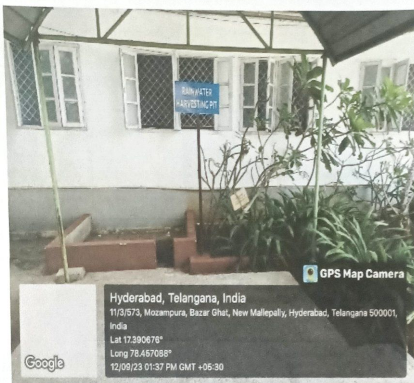
Rain Water Harvesting Facility On The Campus – A Process Of Storing And Purifying Rain Water
