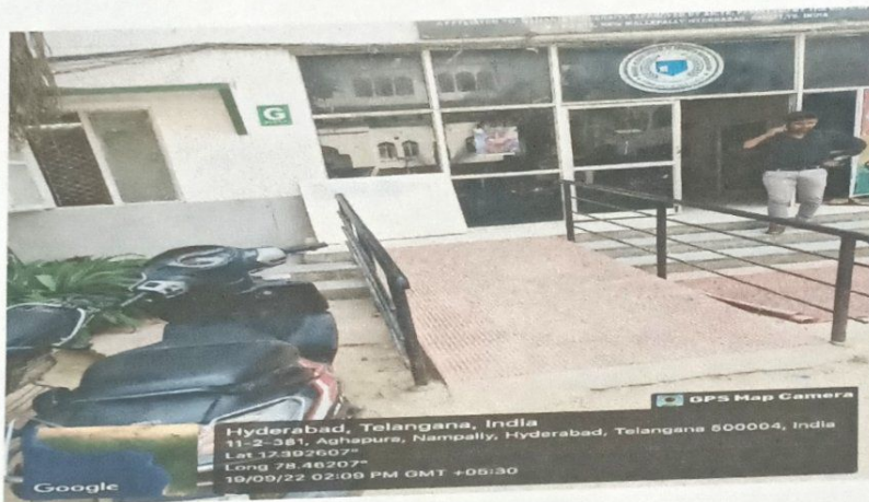
Ramp For Differently -Abled
